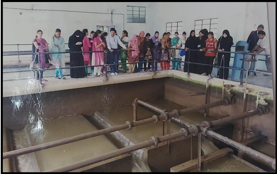
Faculty and Students observed the process of water purification ,at Water Purification Plant, Malegaon
