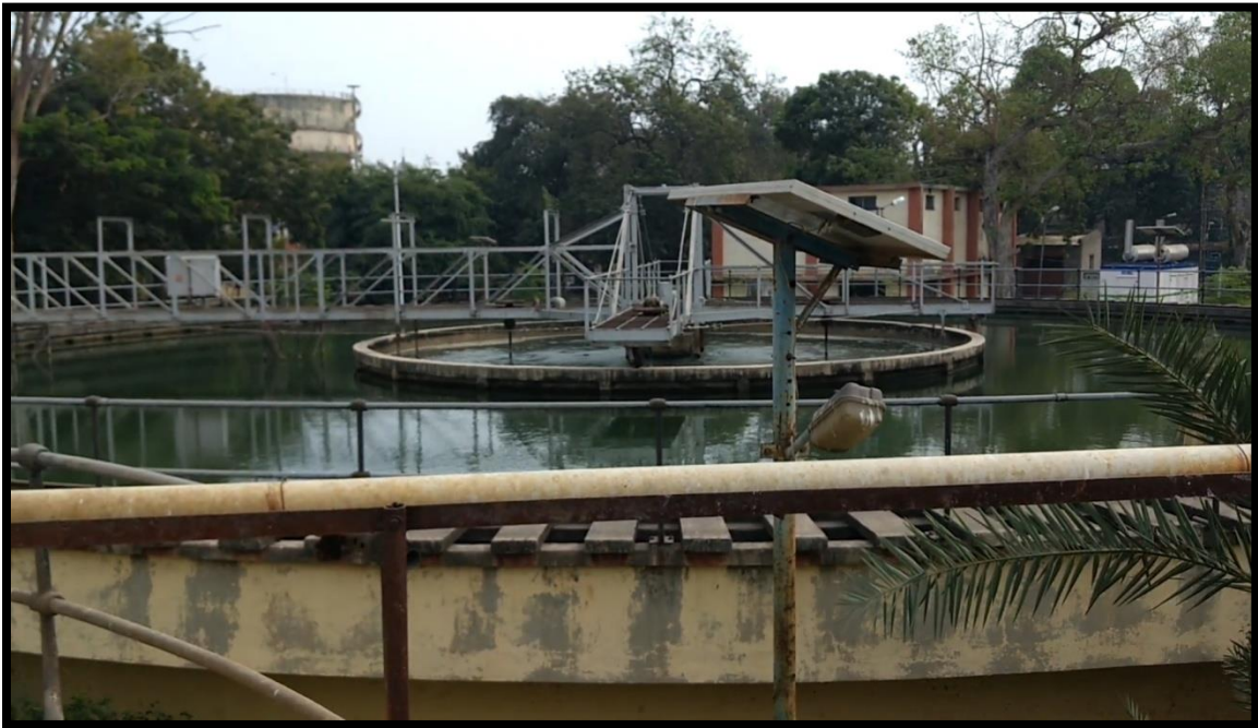
Water Purification Plant, Malegaon
